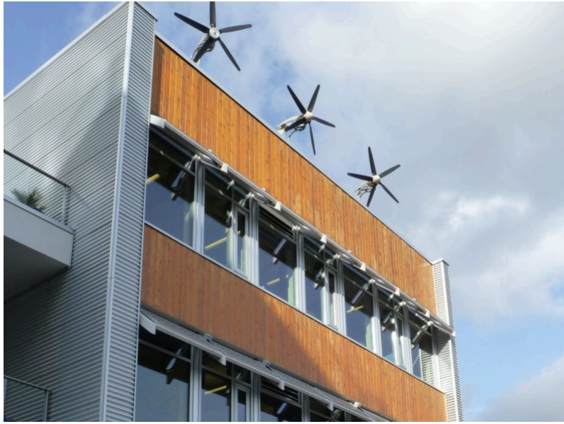
Figure 1.6 Wind power, Dockside Green, Victoria
