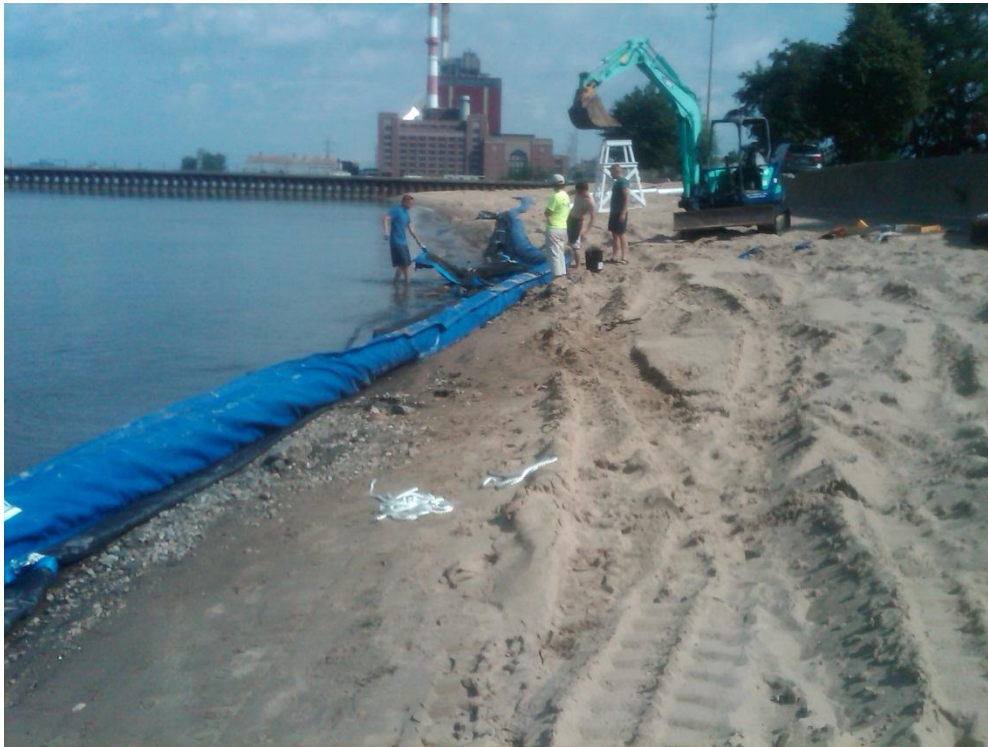
Above: Installation of the barrier in July of 2012.
