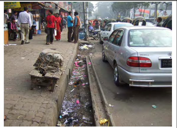
Photo 16.1-1 (4) Obstructions left on Carriageway
