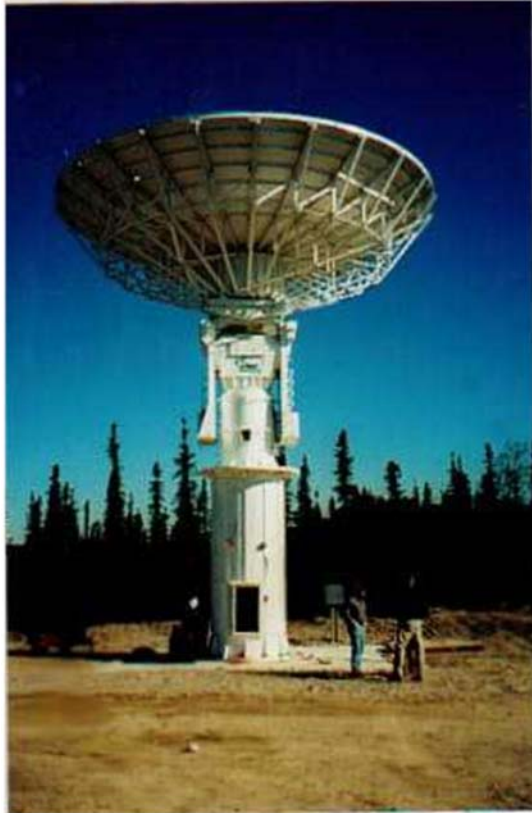
Figure 6-6. USAK05 Antenna before Radome Installation
