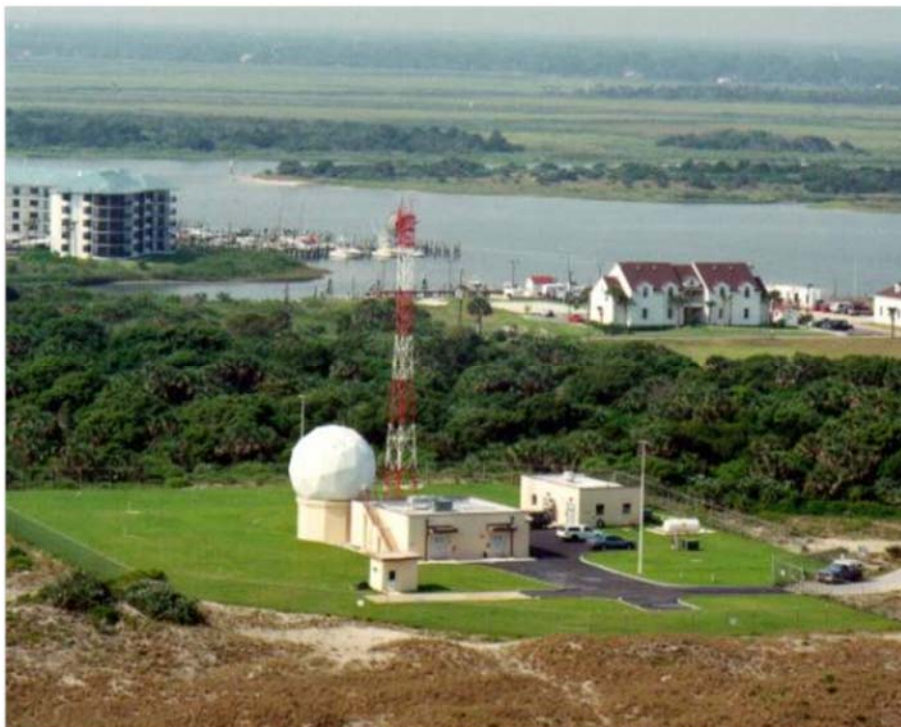
Figure 8-2. PDL Ground Station
