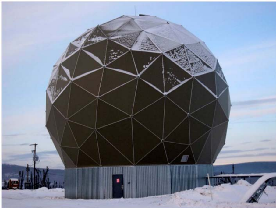
Figure 6-5. USAK05 Antenna Radome
