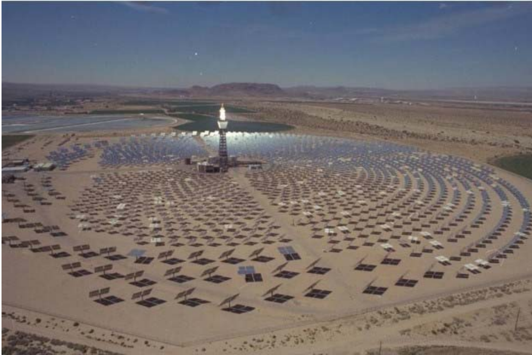
Figure 23: The Solar Two CRS in Barstow (California, U.S.A.) (Courtesy of Sandia National Laboratories)
