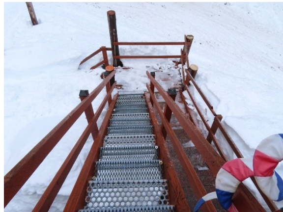
West Fire Escape
