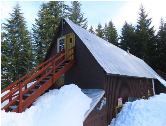
West Side of the Lodge
