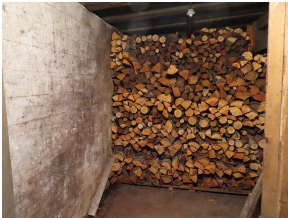
Lower-Level Wood Storage Area
