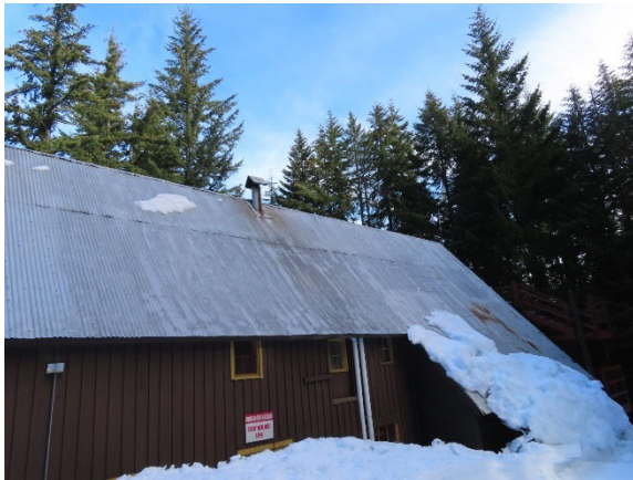
Metal Roof on Lodge
