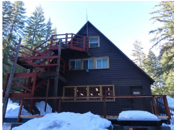
East Side of the Lodge
