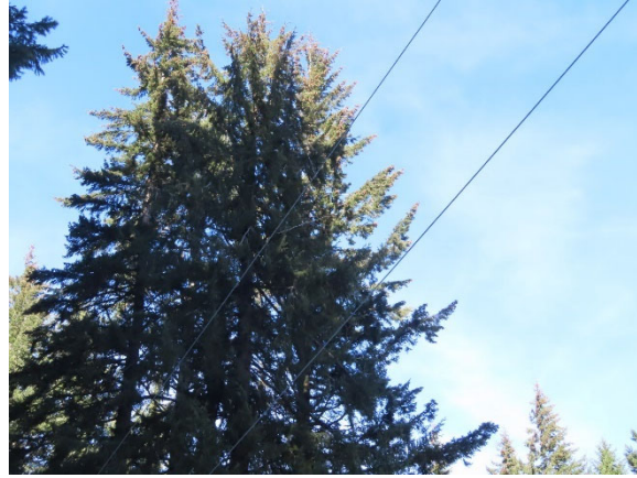
Incoming Electrical Line
