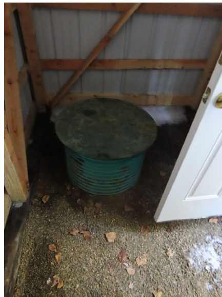
Riser for Buried 1,500-gallon Cistern
