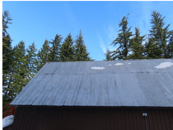
Metal Roof on Lodge
