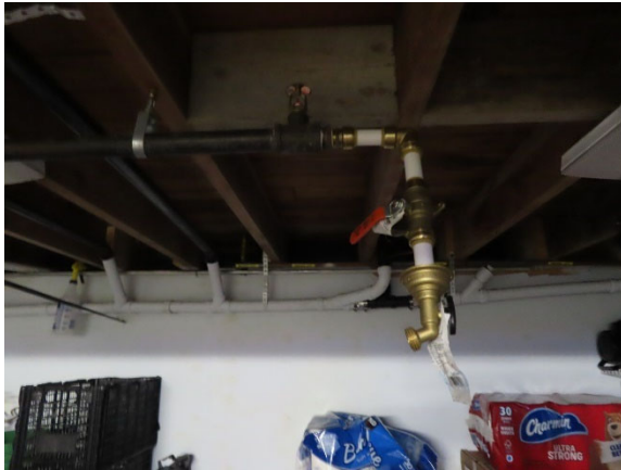
Typical Fire Sprinkler Head
