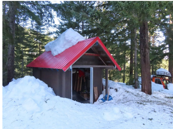
Typical Metal Roof on Outbuilding
