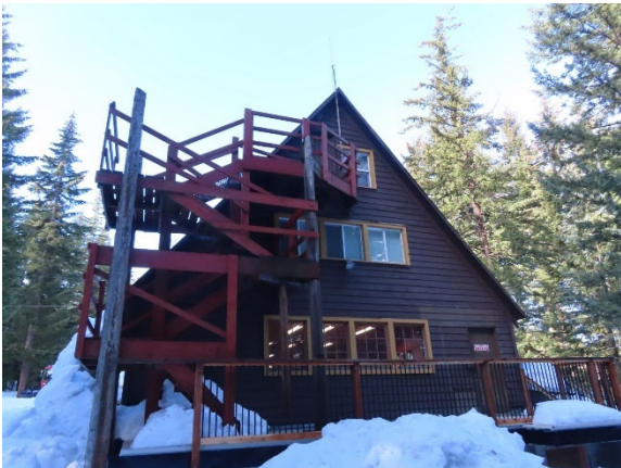
East Side of the Lodge
