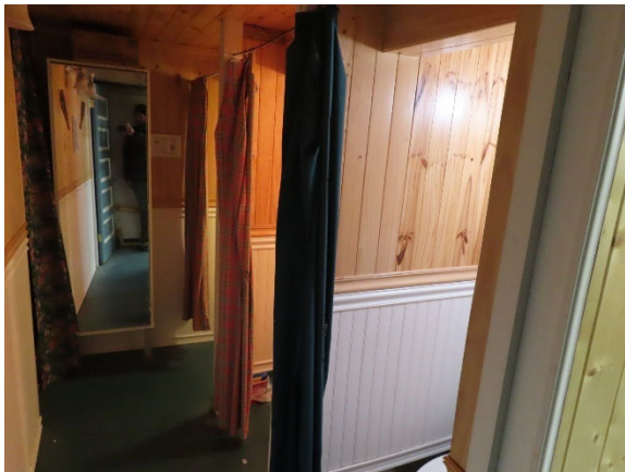
Women's Lower-Level Bathroom
