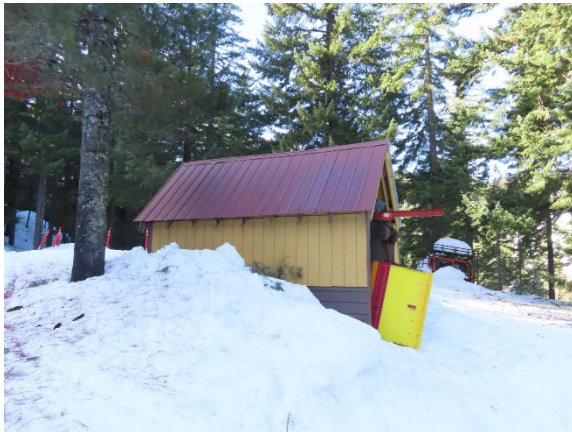
Typical Metal Roof on Outbuilding
