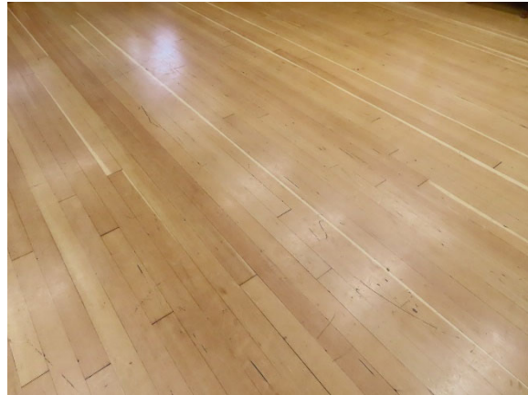
Second-Floor Hardwood Floor
