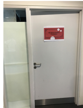
Room Doors (Levels 2 and 3)
