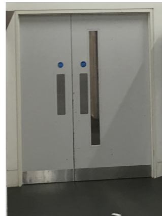
Corridor Doors (Levels 2 and 3)
