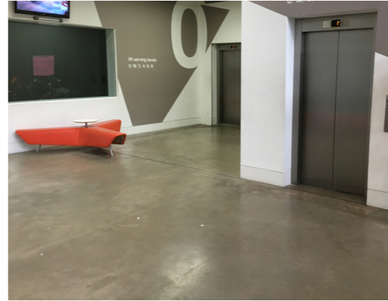
Polished Concrete Floor (Level 0)
