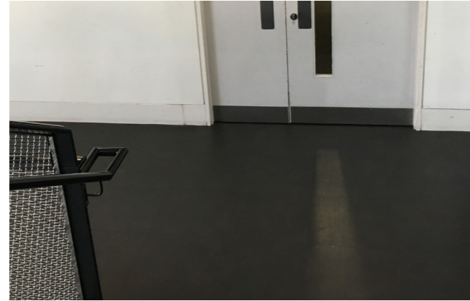
Laminate Floors (Levels M, 2, 3, 5, 7, 9)
