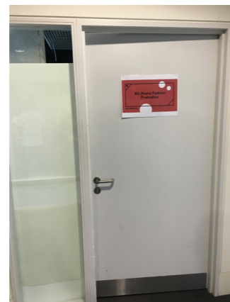
Room Doors (Levels 2 and 3)
