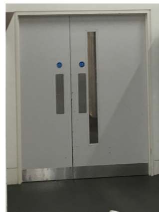
Corridor Doors (Levels 2 and 3)
