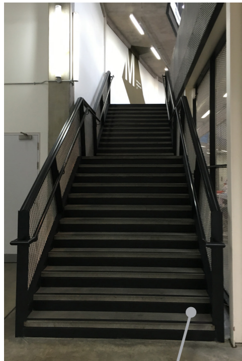
Stairs (Stair Faces)
