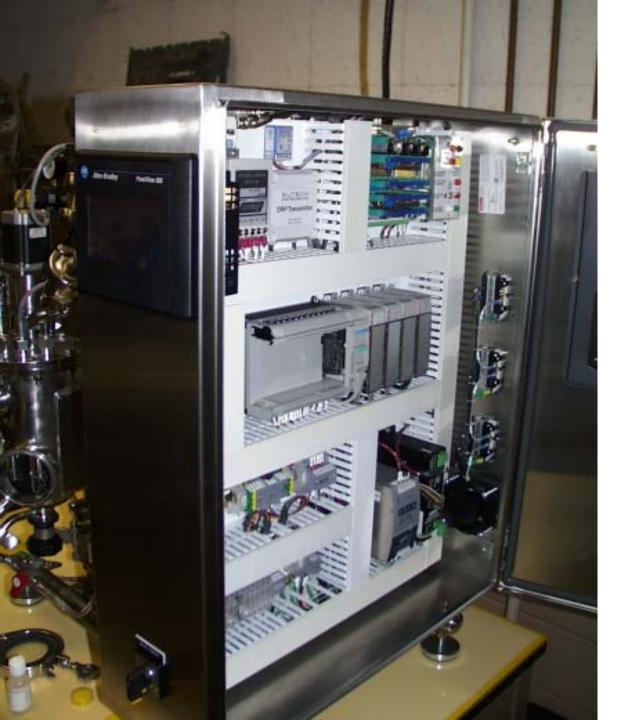
The back view of this reactor, tightly packed with controlling devices and microprocessors, shown in the next picture.
