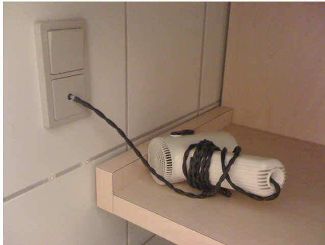
Figure 1.3 In a cheap hotel room, you might find a hair dryer wired directly into the wall outlet. This is equivalent to using the common practice of writing tightly coupled code.
