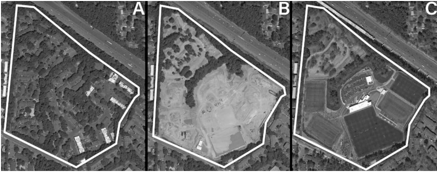
FIGURE 7.2 (A) Flagstone Village and Woodlands Park apartments, May 5, 2014. (B) After demolition, May 7, 2016. (C) Training complex for Atlanta United FC, March 31, 2017. Imagery from Google Earth. Marietta, GA. 33°56′06.14″N 84°29′54.72″W, Eye alt 4122 feet. Image Landsat/Copernicus. www.earth.google.com (February 18, 2018). Boundary added by first author.
