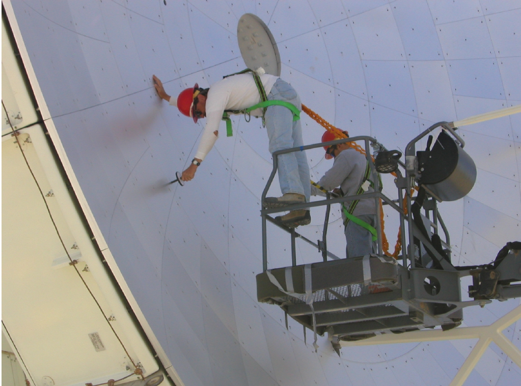
Figure 11: Panel adjustment of the VertexRSI prototype antenna.
