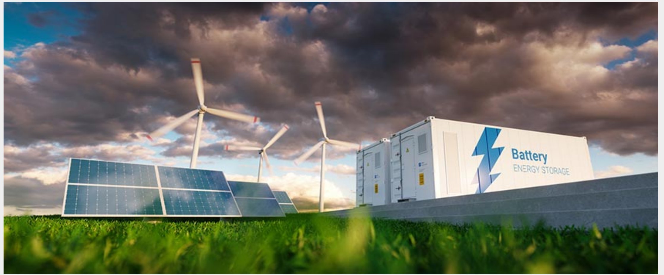
Solar PV and Wind energy Storage (NREL)
