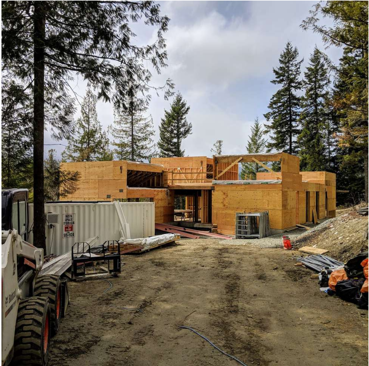
Early framing in year one of construction – 2018
