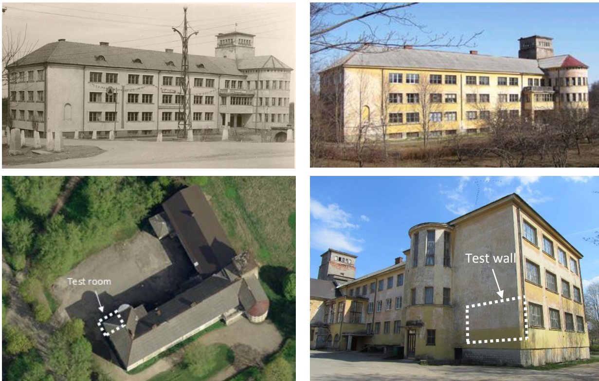
Figure 4.38: Photographs of the building, received from the authors of [Klõšeiko et al. 2015].
