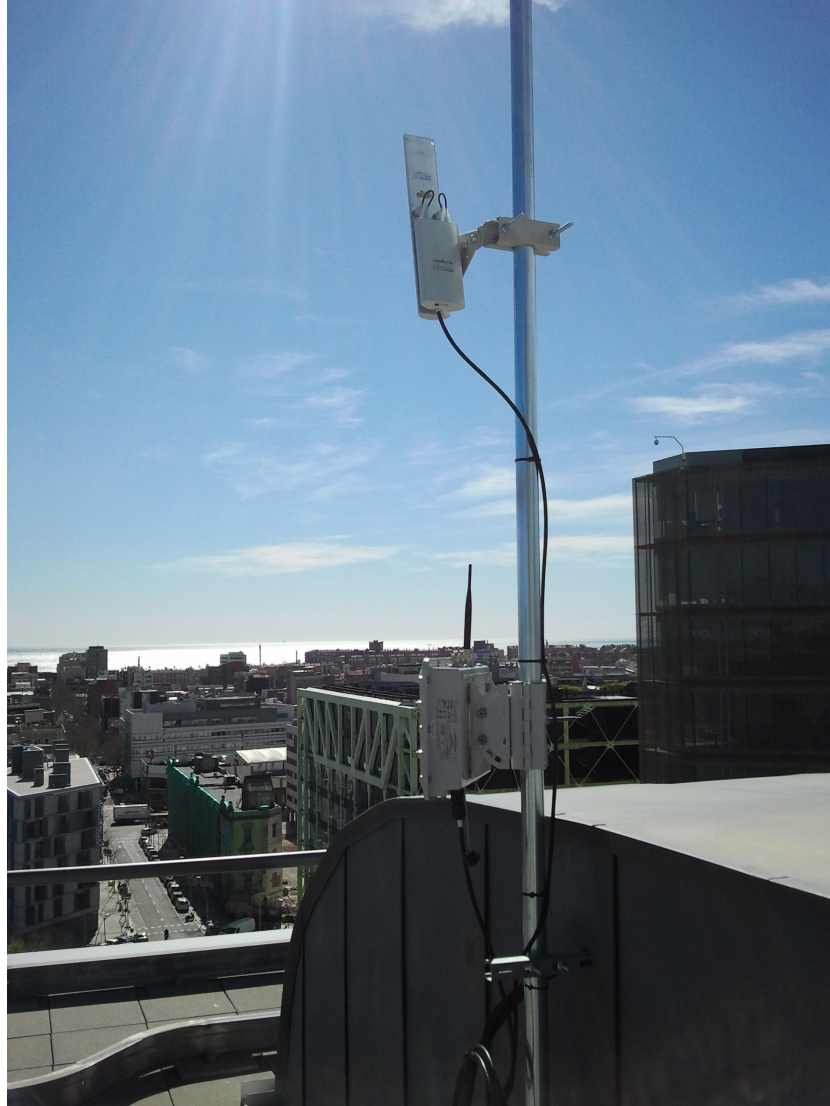
Figure 3.9: Rocket M5 installed on the roof of Roc Boronat Building (2)
