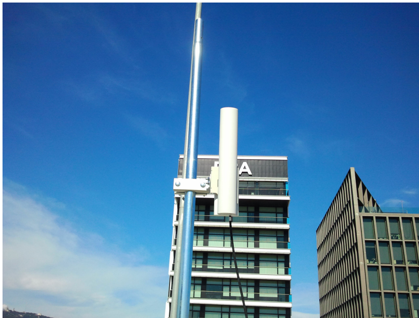
Figure 3.8: Rocket M5 installed on the roof of Roc Boronat Building (1)
