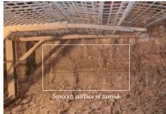
FIGURE 11: Effect of V-cut blasting with auxiliary holes.
