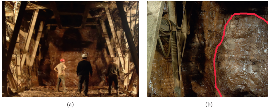
FIGURE 9: Blasting effect of double horizontal V-cut blasting.
