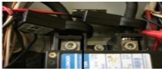
CTs clamped to both phases on the electrical box before the main circuit breaker.
