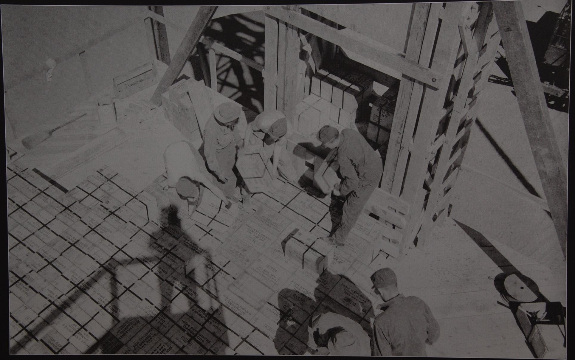
Personnel stack 4,000 boxes of TNT, at 50 pounds a box, to make a stack of 100 tons of TNT for the May 7, 1945, calibration test.
