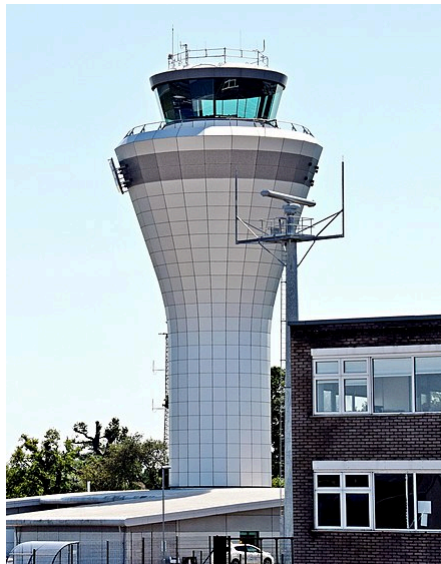
Control tower at Birmingham Airport , England.
