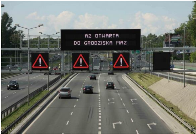
Fig. 3. An example of using intelligent transportation systems for road traffic management through information on variable speed limit signs
