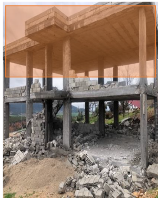
Figure 1: Earthquake-damaged reinforced concrete building.
